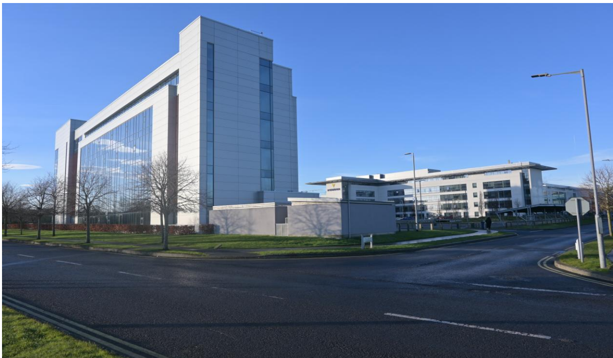
Figure 13.9: The building at the entrance to Airside Business Park
